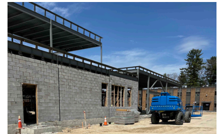
Above: Area B masonry CMU walls being installed.
