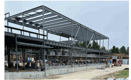
Above: Area B steel detailing continues; masonry CMU walls underway.
